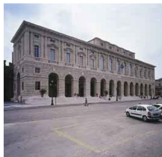
The Palazzo della Gran Guardia, a 17th-century building, is a key element in the scenic plan of Piazza Bra in Verona. The Gran Guardia at present houses a part of Count Giuseppe Panza di Biumo's collection. The Count is portrayed (facing page) by Giorgio Colombo in Bruce Nauman's Green Light corridor , Centro de Arte Reina Sofia, Madrid
